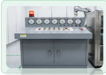
Voltage Test (Under Water)
